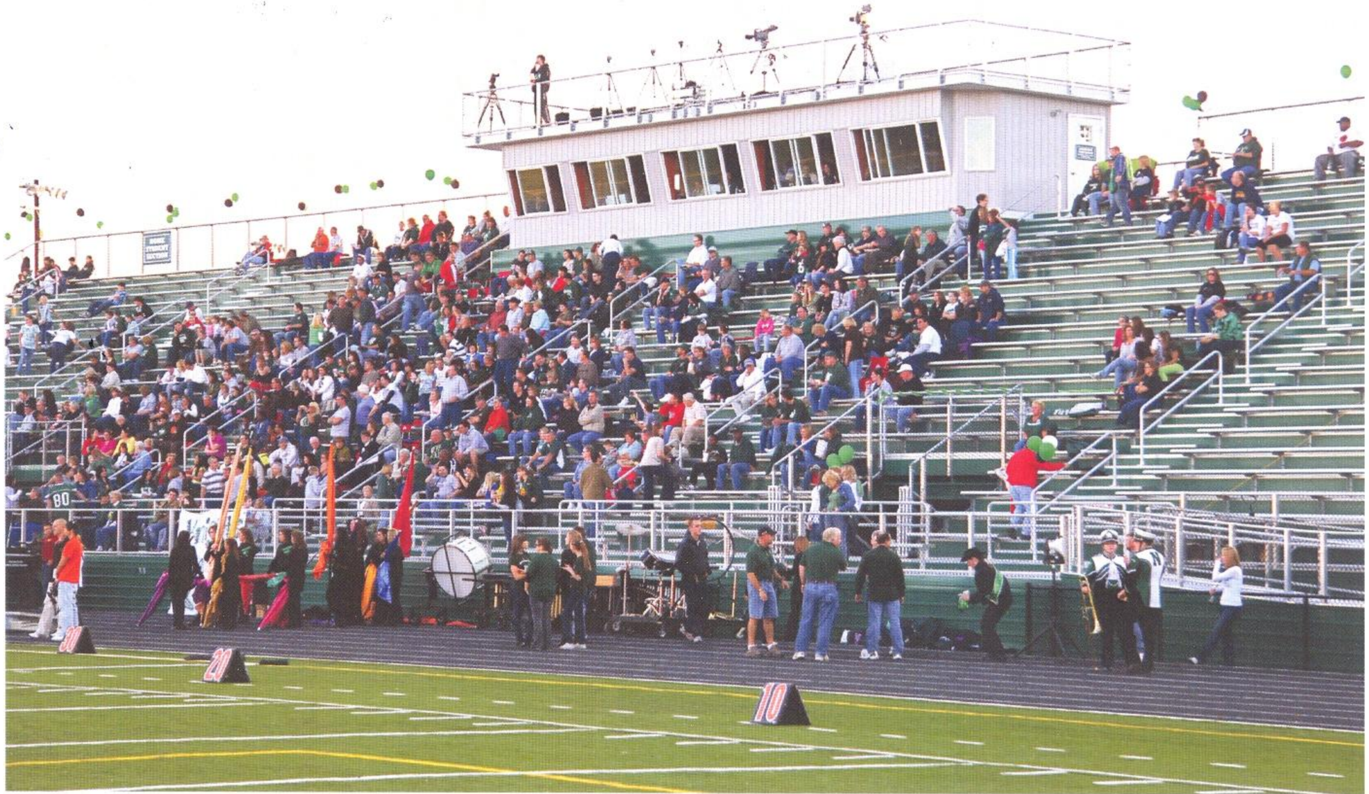
FORWARD PROGRESS As part of the athletic facility upgrades, the new football stadium includes separate locker rooms and concession stands for both home and visiting teams, low maintenance aluminum bleachers and a new press-box.
